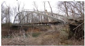
The Springfield Bridge was built in 1874 by the King Bridge Manufactory and Iron Works of Iola, Kansas. It was shipped disassembled, then erected on footings built by a local mason. The bridge was an essential link in an historic route connecting Des Arc on the White River with Springfield, the onetime seat of Conway County. The Springfield bridge is a good example of the now-rare bowstring truss design, as well as the oldest surviving highway bridge in the state.
